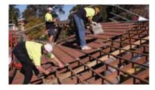
2. Remove old tiles & battens All the old tiles, ridges and battens are removed. Care is taken over existing ceilings and fixtures.
