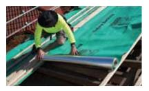
**3. Install Sarking\*** Sarking provides insulation and reflects up to 95% of radiant heat entering the roof.
