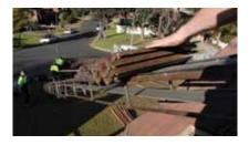
**5.** Load up new tiles The new roof tiles are sent up to the roof using a conveyer system.
