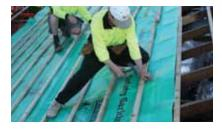
**4. Install new battens** New battens are installed ready for the new roof tiles to be laid.
