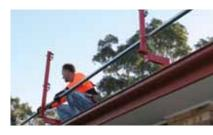
**1. Install Safety Rail if required** Safety is a priority. Guardrail is installed around the perimeter of the roof to prevent roof tilers from falling and to keep your family safe.
