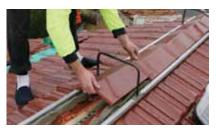
7. Ridge tiles installed Ridge tiles are installed and bedded in place using mortar.
